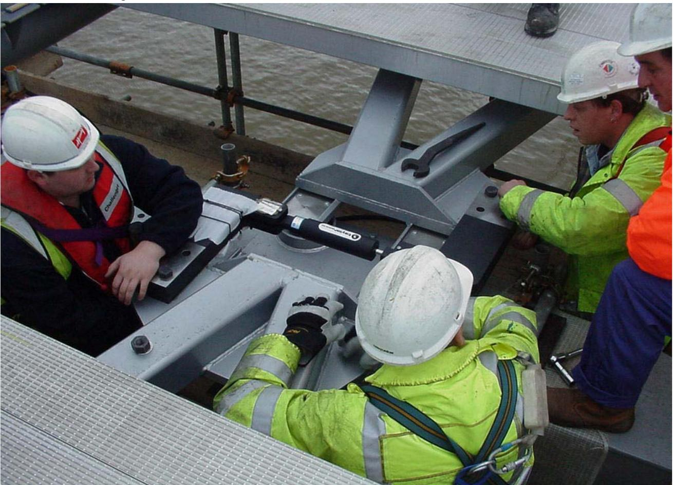
**Figure 3. Viscous damper being fitted between chevron braces beneath the deck**
