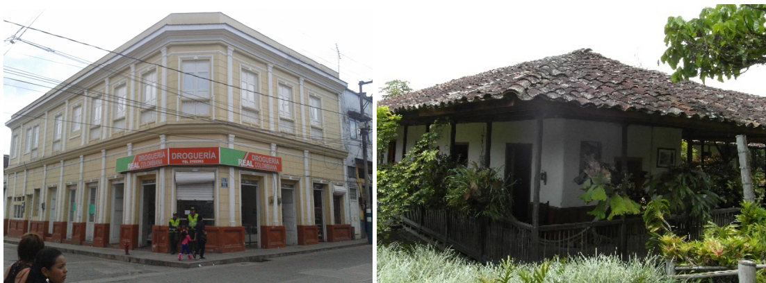
Figure 1. Traditional urban and rural bahareque housing in Colombia: (L) Sevilla (Lopez, 2016); (R) Armenia (Kaminski, 2016).
