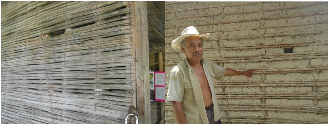
Figure 3. Typical wall matrices for traditional bahareque (Kaminski, 2016): (L) esterilla/caña picada (sheets of bamboo formed by splitting bamboo along its length and then unrolling it; (R) caña brava/vara de castilla (small diameter bamboo/cane).
