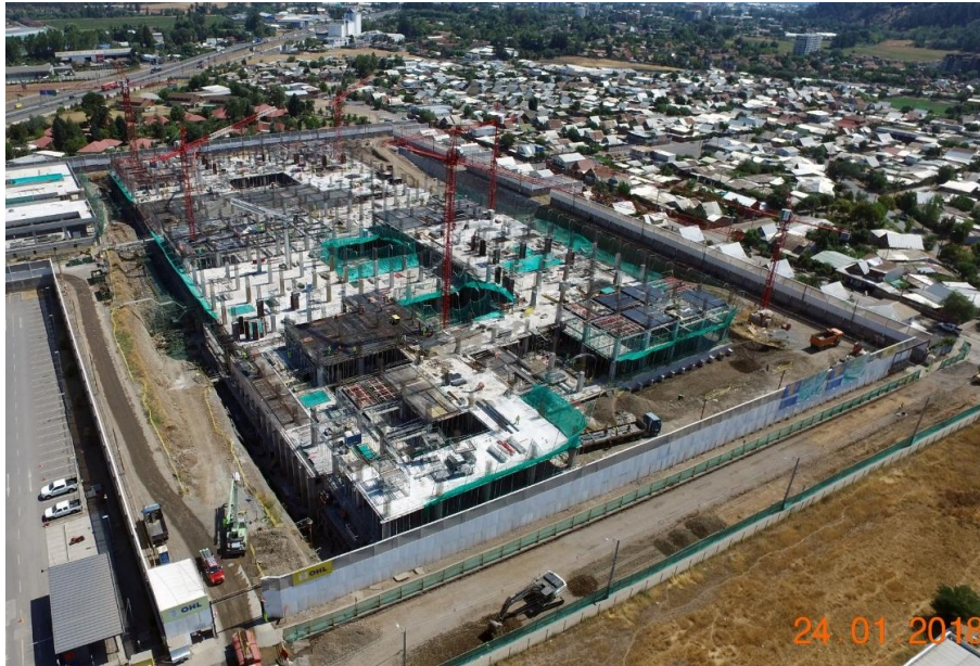
Figure 2. Hospital de Curicó erection
