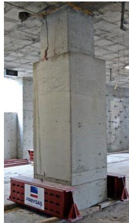
Figure 19. Marmara: Column before the installation
