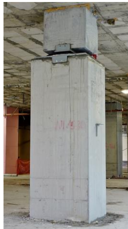
Figure 22. Marmara: Column after the installation
