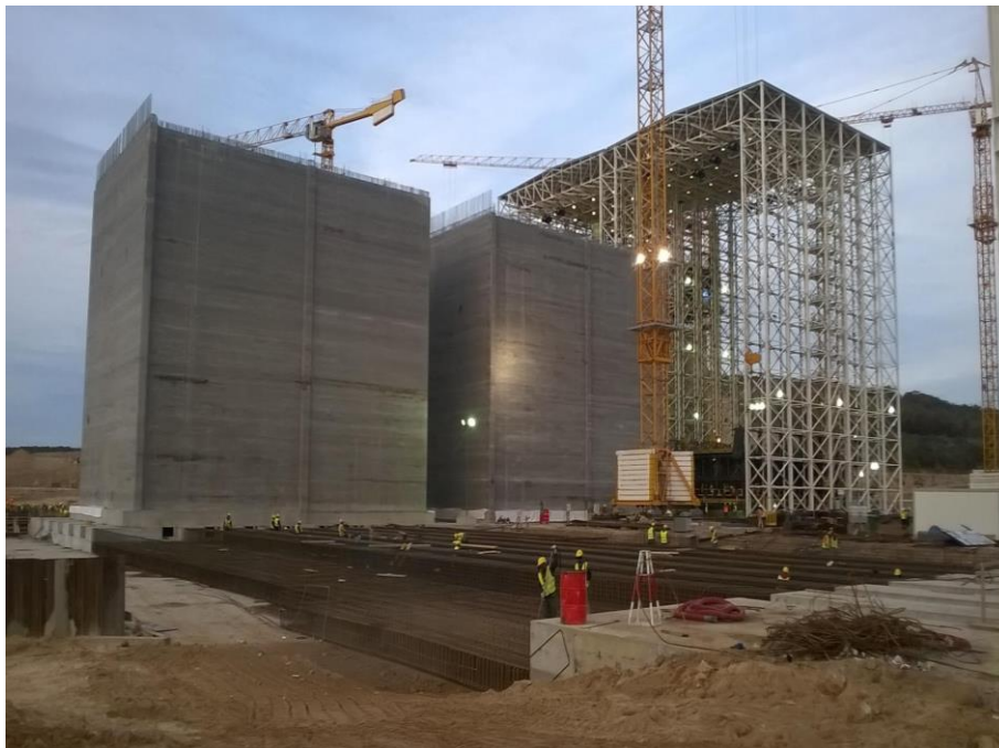
Figure 11. Construction of breakwater caissons under way.
