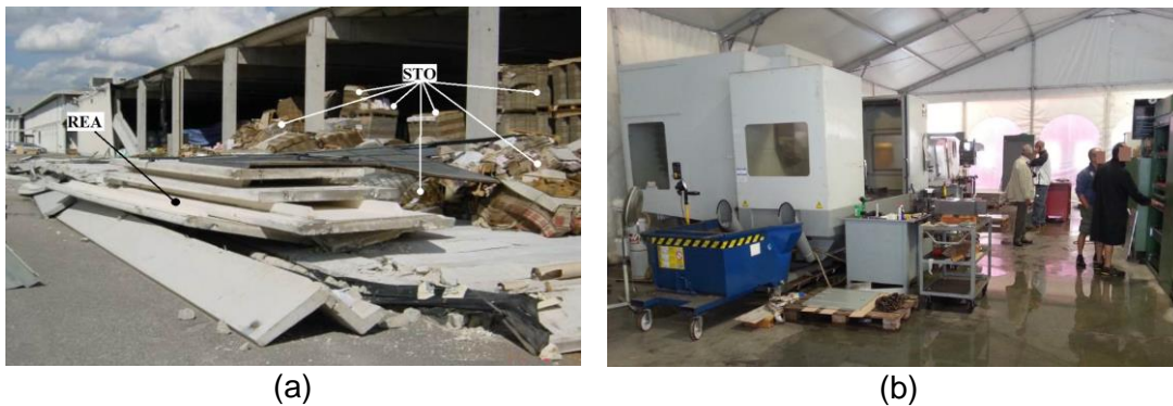
Figure 3. Examples of consequences after the 2012 Emilia earthquake (a) REA and STO (b) REL (source: Agenzia regionale per la ricostruzione – Sisma 2012).
