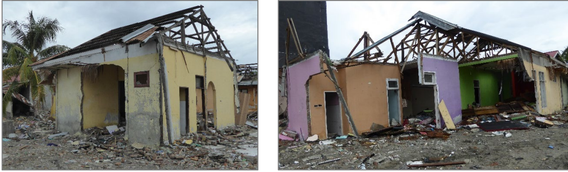
Figure 10. Heavily damaged CM houses in Palu bay area along the Jl. Rajamoili road, about 100m from coastline. The walls of this house were directly hit by the tsunami inundation.
