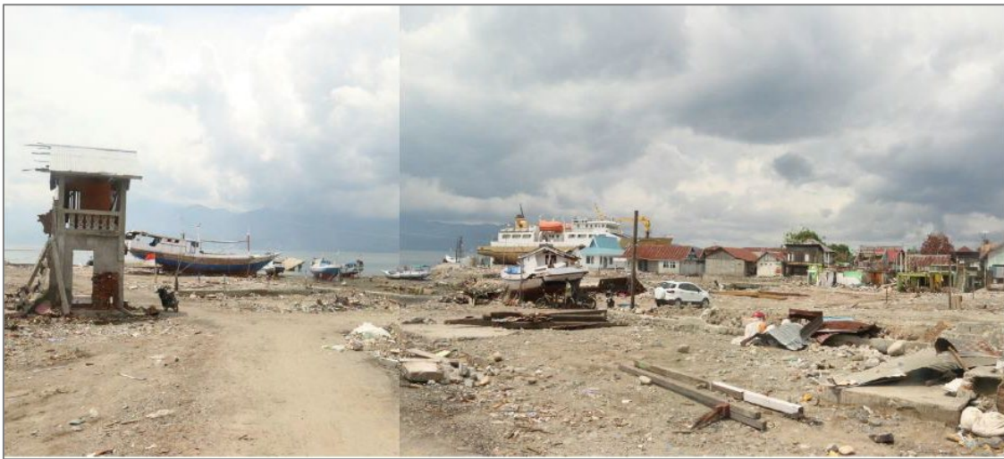
Figure 9. Wani village on the east coast of Palu bay which experienced considerable damage.
