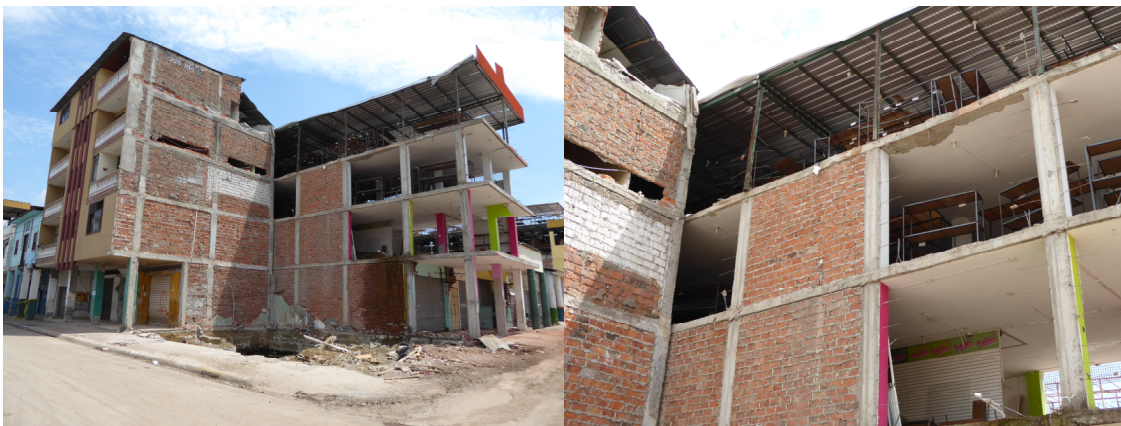
Figures 1 and 2. Typical low-rise RC frame with masonry infill.
