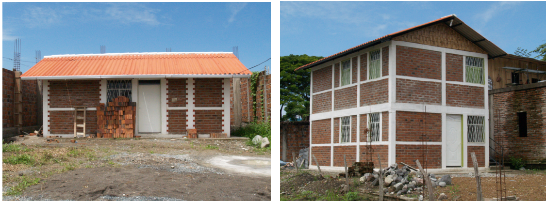
Figures 17 and 18. A one and two-storey CM house built by ECOSUR in Pedernales in 2017.
