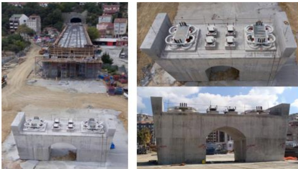
Figure 7. Views of Alibeyköy viaduct under construction.
